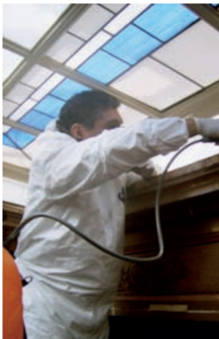
Aspirando paneles in situ .
